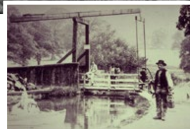
The Canal bridge at Talybont
